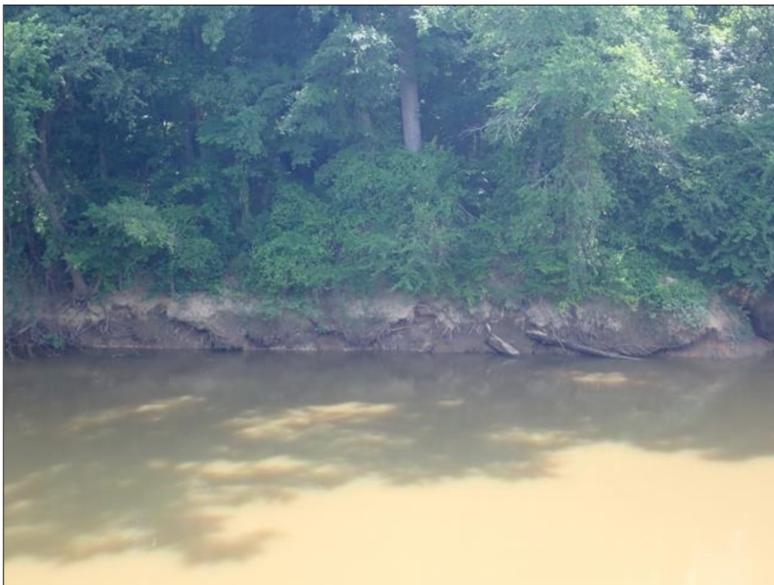
along channel embankments, vertical cuts (up to 4 foot high)
