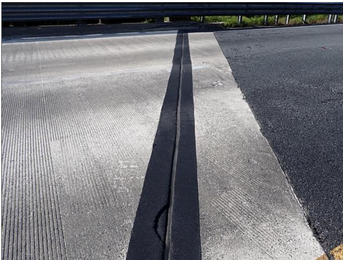
end bent 1 joint
