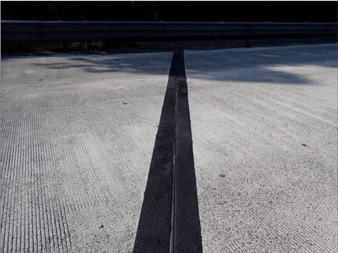
end bent 2 joint
