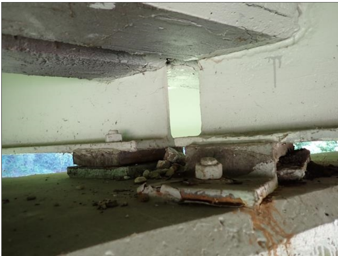
interior bearing assembly
