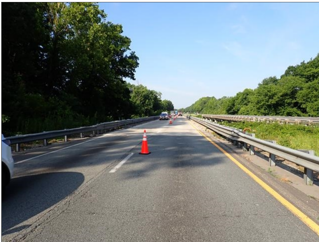
north approach looking south
