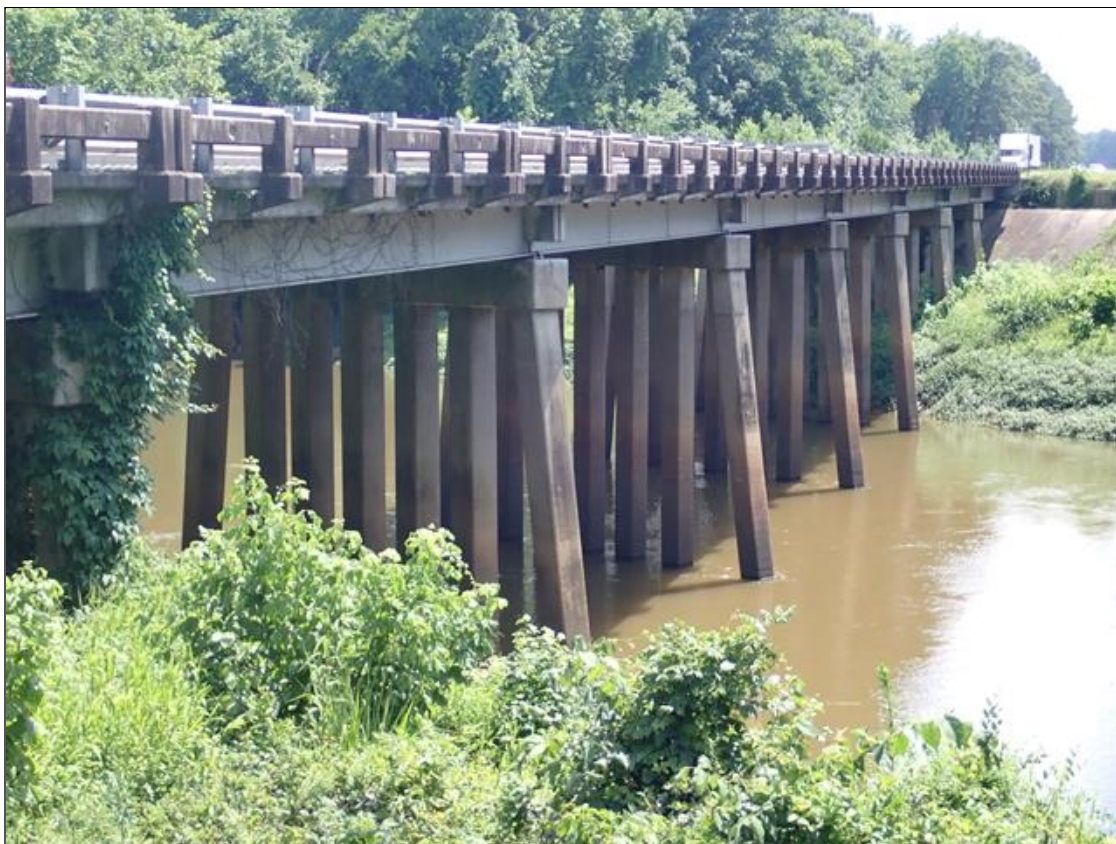
upstream profile looking east
