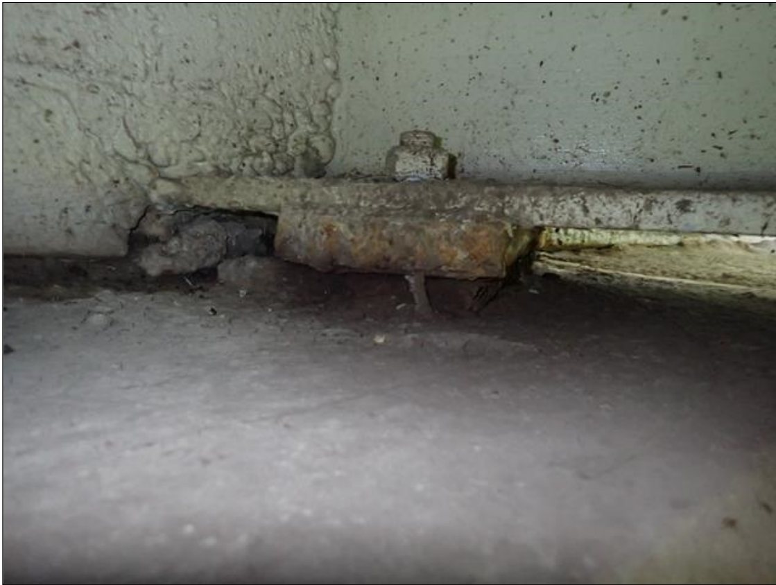
end bearing assembly
