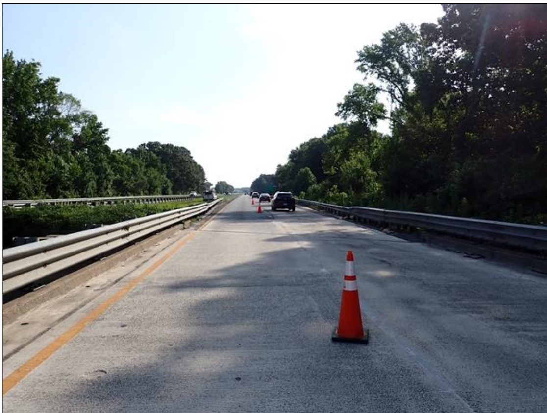
north approach looking north
