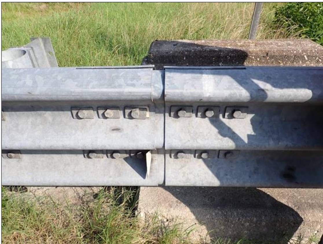
southwest guardrail attachment
