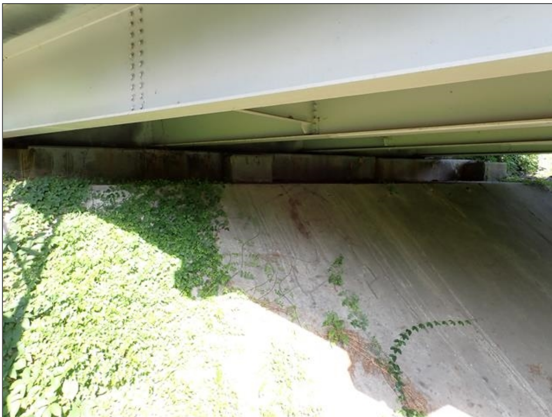
end bent 2 and slope protection
