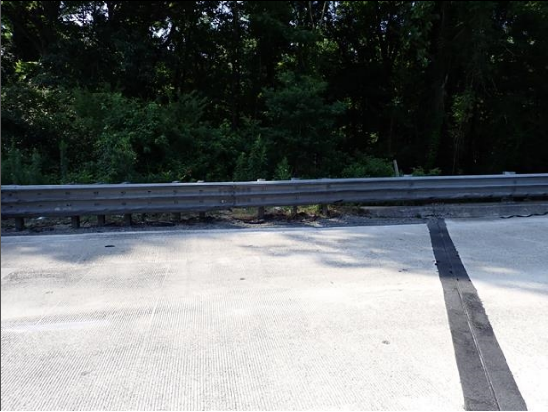
northeast guardrail attachment
