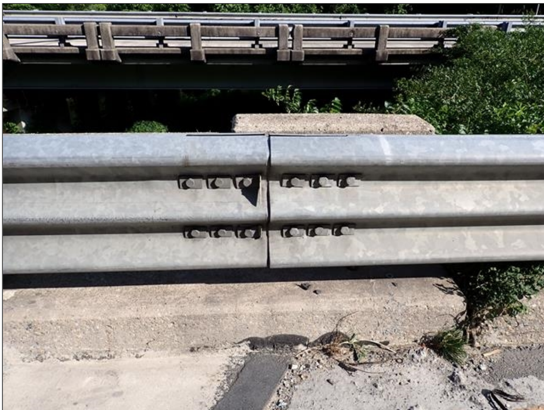
northwest guardrail attachment
