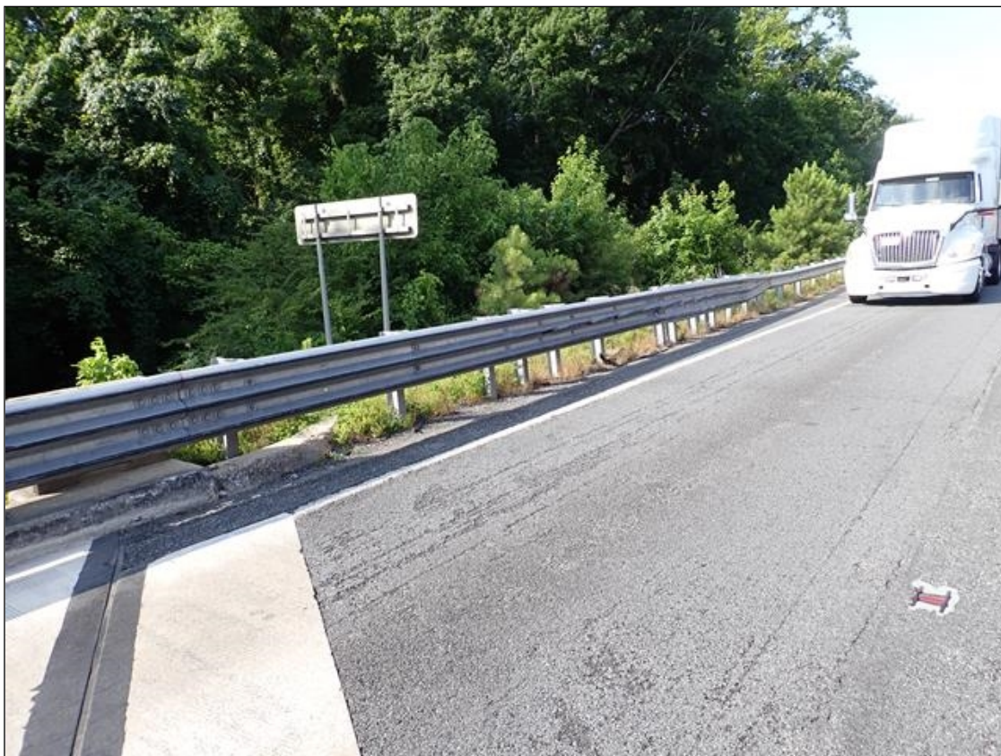
southeast guardrail transition
