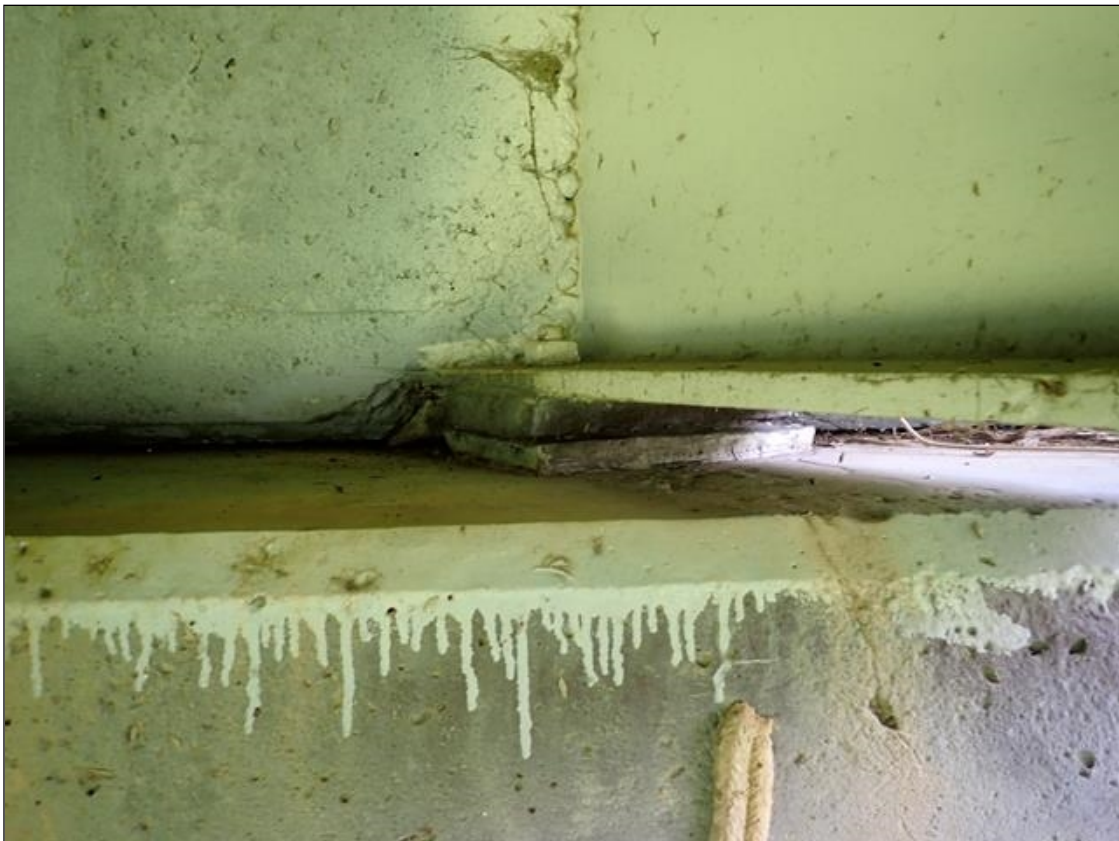
end bearing assembly
