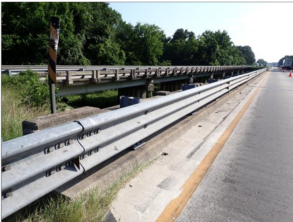
left bridge rail
