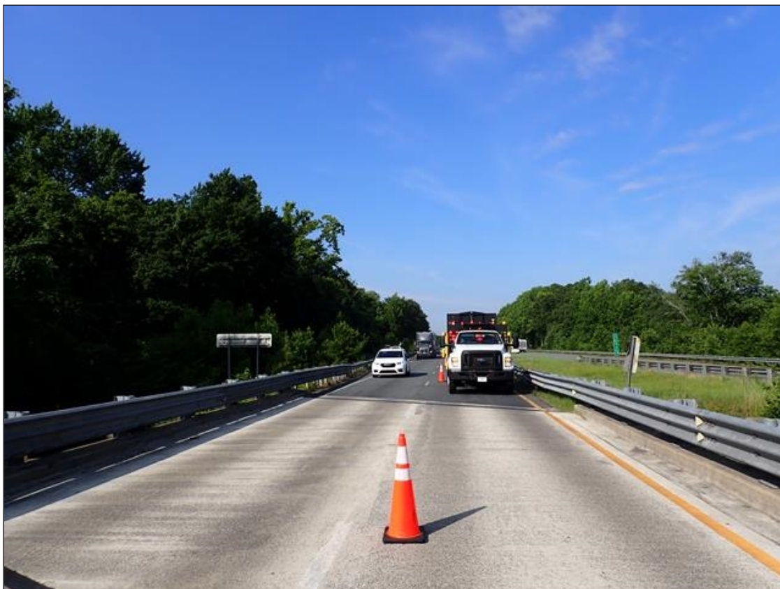
south approach looking south
