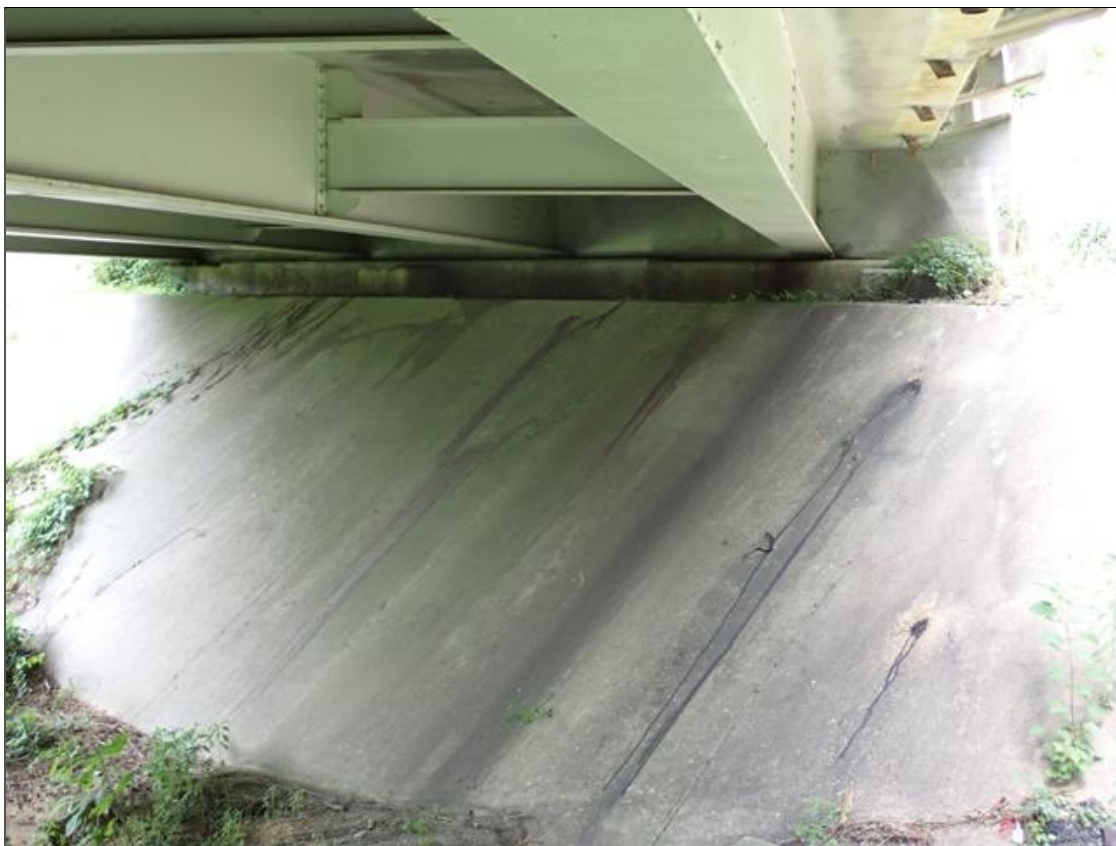
end bent 2 and slope protection
