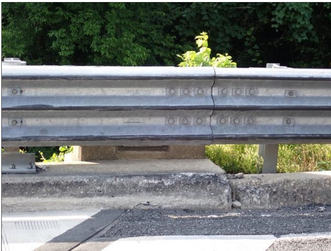
southeast guardrail attachment
