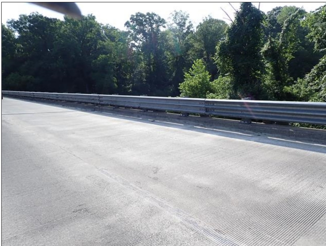
right bridge rail
