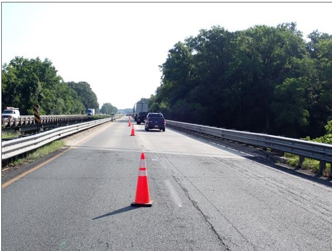
south approach looking north
